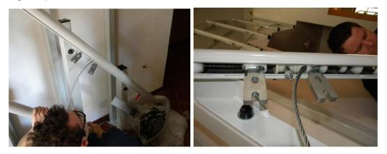
• Add the drive wheel cover and the mains filter again onto the drive wheel. This cover must be fixed before the rope is tensioned!
