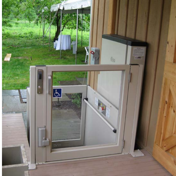
Upper level gate with optional glass inserts
